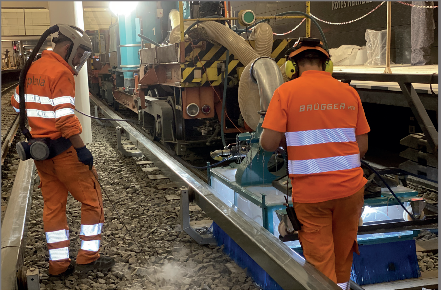
Picture: Fine dust cleaning Subway tunnel Berlin DE
