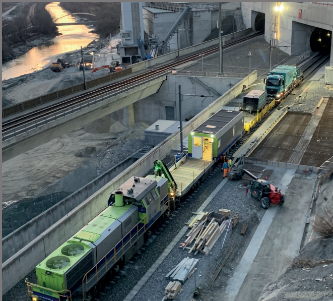
Picture: Cleaning train Lötschberg base tunnel south portal
